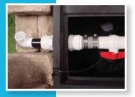
When the basin is placed below the spout, the pump will be connected to a hose that feeds the water up to the spout and catches it to recirculate.
