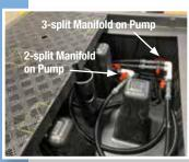
Check These Pump Assemblies should be under the Pump Access, and the PVC Center Support Column should be in the center of the basin.
