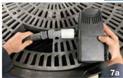
**7b** Set attached pump and hose in the basin. This fountain pump should be located beneath the pump access panel and inside the fountain basin with the pump positioned as close to the pump access opening as possible for best accessibility.
